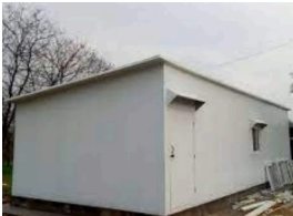
Rest Room Talegaon Pune
